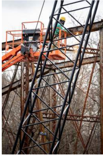
A construction worker cuts a beam of the Kelly Road bridge Tuesday as the bridge is disassembled for removal.
