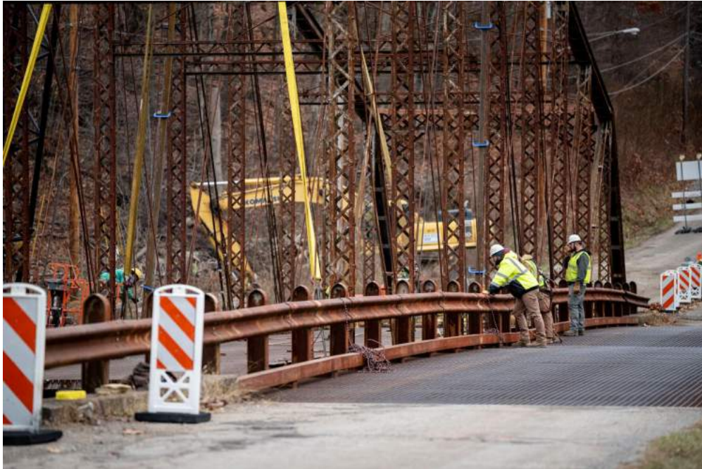
A construction crew works on deconstructing the Kelly Road bridge Tuesday in Sharpsville. A newer bridge adjacent to the metal bridge that has been used for all traffic in recent years will remain until half of a new bridge is built.
