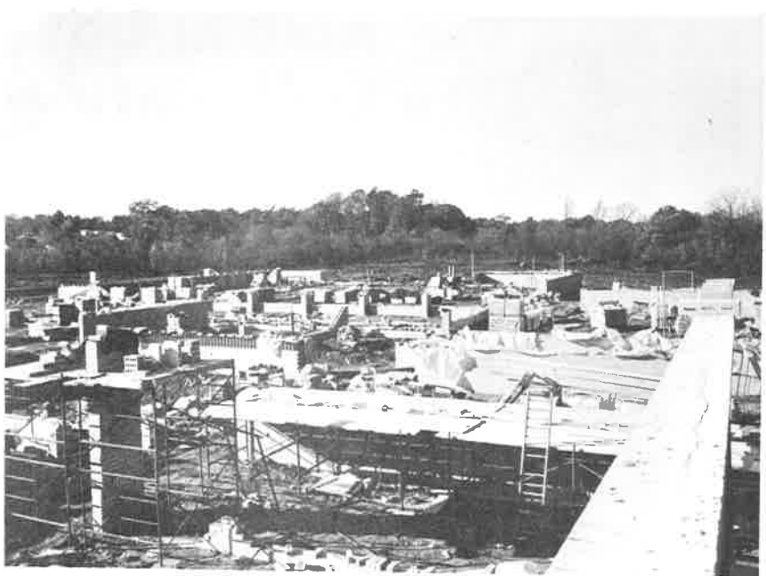
Fifth and sixth grade students will enter the new elementary school for the first time next fall. Construction on the $13 million school started last April. The building includes 22 classrooms, music, art, special education, and lecture rooms, cafeteria, a multi-purpose room, and extensive instructional materials facilities to be used as a center for all the elementary libraries.
